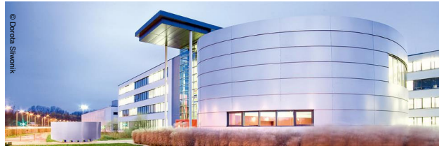
Hannover Center for Production Technology (PZH) opened in 2014
